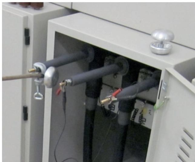
➤ Encapsulated substation, access from front busbar
